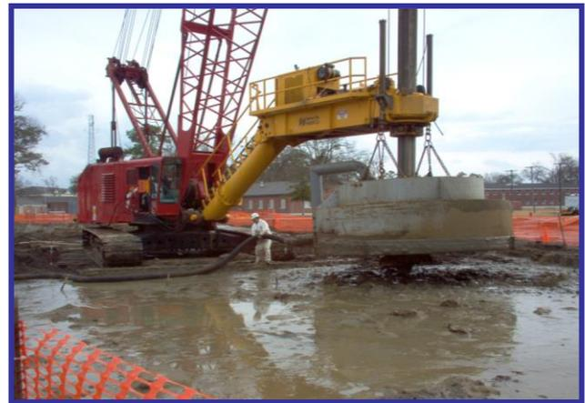
*Site 88 soil mixing with ZVI-clay addition. Soil was mixed with zero valent iron and clay to treat and bind contaminants, resulting in 92% contaminant reduction, equivalent to 26,000 pounds of solvent.*
